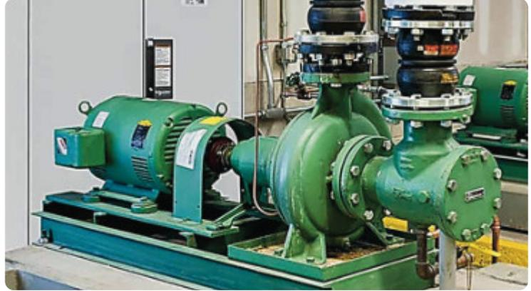
Misalignment is critical in direct coupled machines (with coupling)
