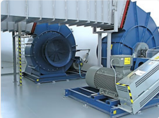
Unbalance is critical in fan installations (direct coupled or with belt pulley transmission)
