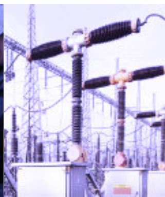
CORONA, PARTIAL DISCHARGE DETECTION
